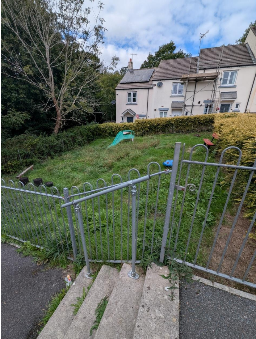
Path and steps leading to entrance gate
